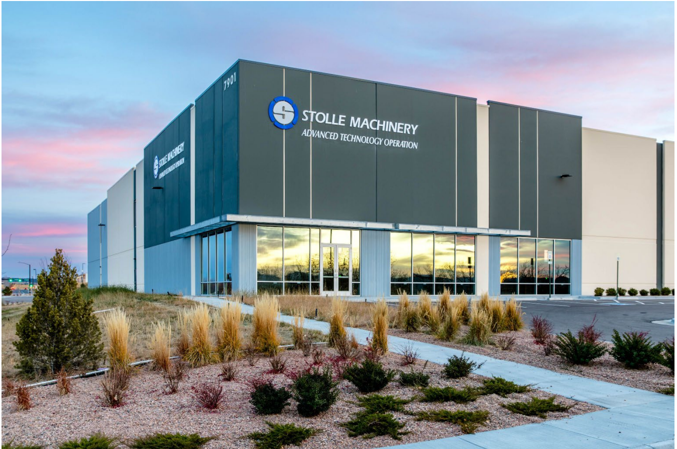
New Stolle Advanced Technology Operation (SATO) in Centennial, Colorado, USA
